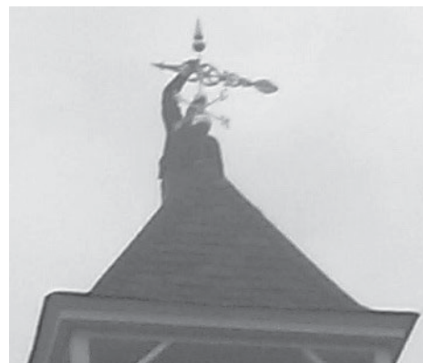
Scot Schwartz of R&R Roofing places the weathervane on Town Hall.
